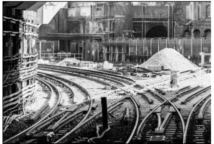
Two views looking east at Farringdon from the westbound platform on 16 February 2017 ( Left ) showing the new westbound points and on 15 March 2017 ( Right ) after the eastbound points had been installed and commissioned.
