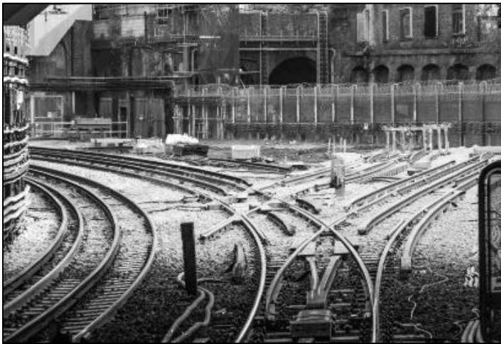
Two views looking east at Farringdon from the westbound platform on 16 February 2017 ( Left ) showing the new westbound points and on 15 March 2017 ( Right ) after the eastbound points had been installed and commissioned.
